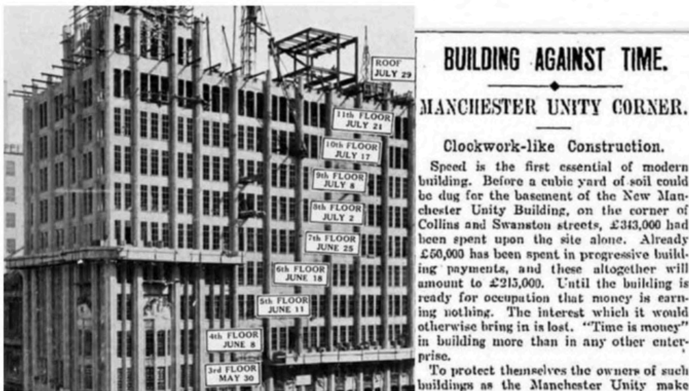
📷 The remarkable building schedule for the Manchester Unity project and, right, a 1932 newspaper article about the speed of construction. Picture: Trove
